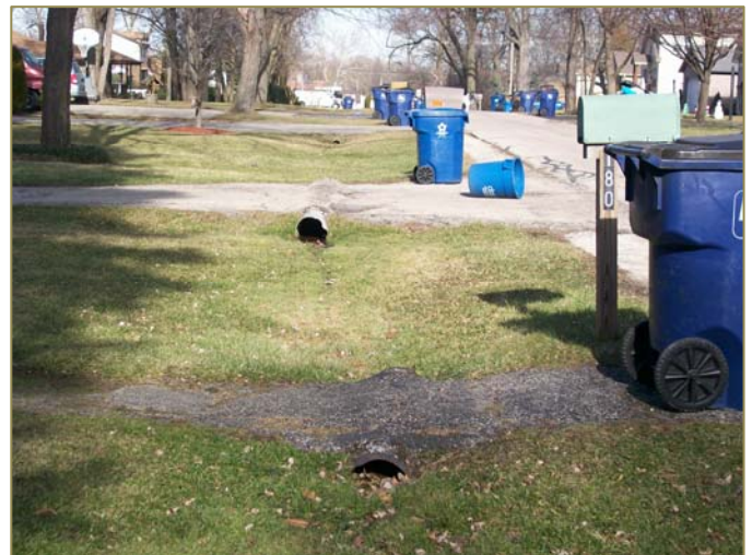
Water must travel through a series of deteriorated culverts before reaching the outfall.
