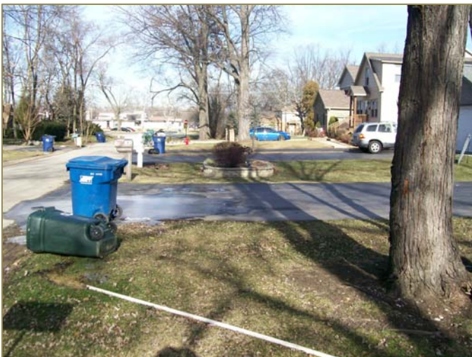
Residential sump lines currently flow above ground. Currently, slopes of the open drainage system are insufficient for proper drainage.
