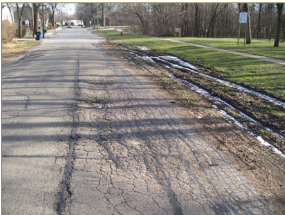
This deteriorated section of roadway along Wood Avenue may require significant undercut.
