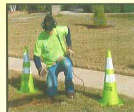
Step 1. Leak Detection
