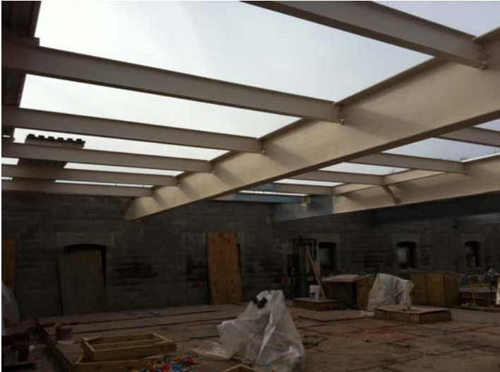
Madison Coatings began applying L69F Epoxoline paint system to the structural steel members throughout the Tertiary Filter Building
