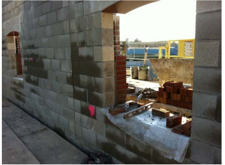
Bos & Son began laying face brick and chiseled-face units at the window openings in the Tertiary Filter Building south wall
