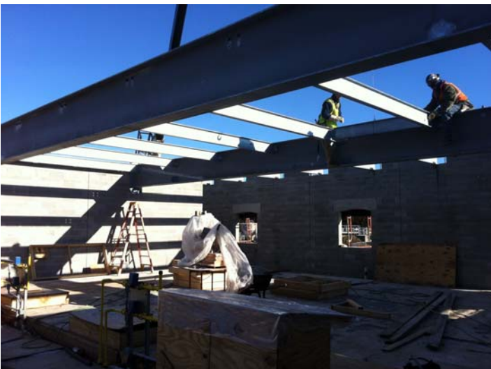
Area Erectors began setting W30 structural steel members, followed by W10 cross-members at the Tertiary Filter Building
