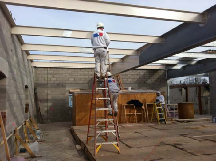
Madison Coatings began applying L69F Epoxoline paint system to the structural steel members throughout the Tertiary Filter Building
