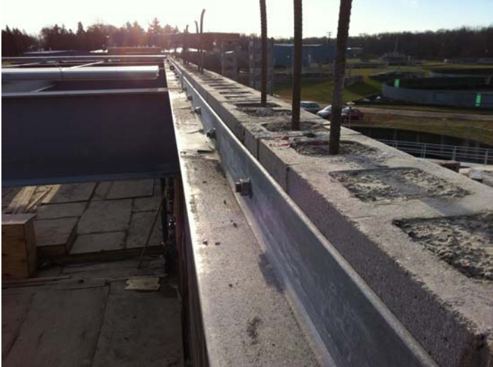
Area Erectors installed roof deck support angles around TFB
