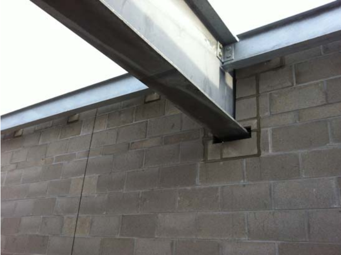
Bos laid partial masonry blocks around beam penetrations
