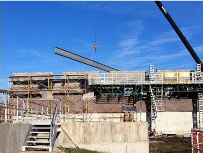
Area Erectors began setting W30 structural steel members, followed by W10 cross-members at the Tertiary Filter Building
