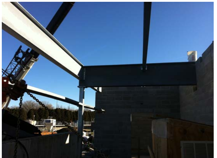
Area Erectors began setting W30 structural steel members, followed by W10 cross-members at the Tertiary Filter Building
