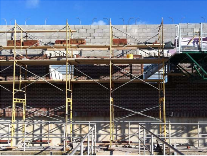
Bos & Son began laying face brick and chiseled-face units at the window openings in the Tertiary Filter Building south wall
