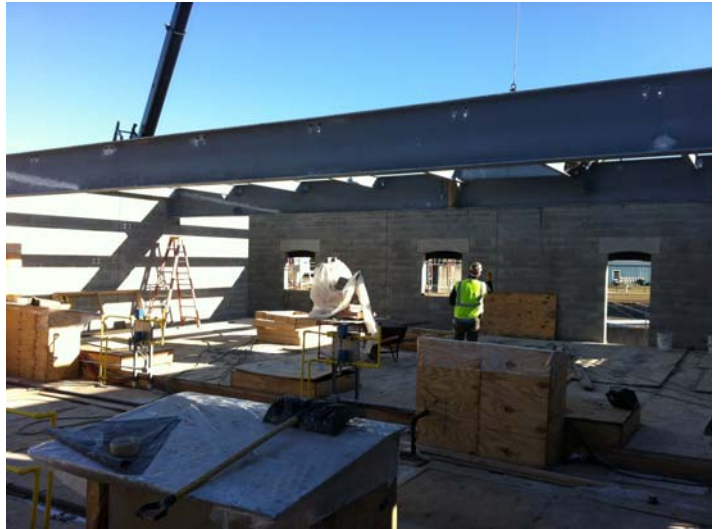
Area Erectors began setting W30 structural steel members, followed by W10 cross-members at the Tertiary Filter Building
