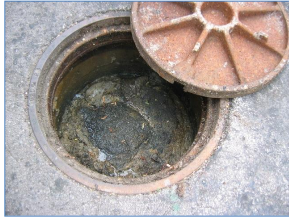
Grease found in Bensenville Manhole
