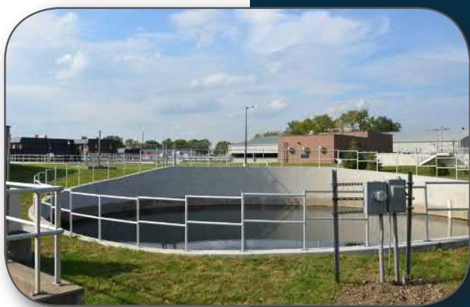
**8 EXCESS FLOW AND FLOW EQUALIZATION TANK**—Excess flow is diverted to an excess flow and flow equalization tank. This tank allows temporary storage and partial treatment during wet weather events.
