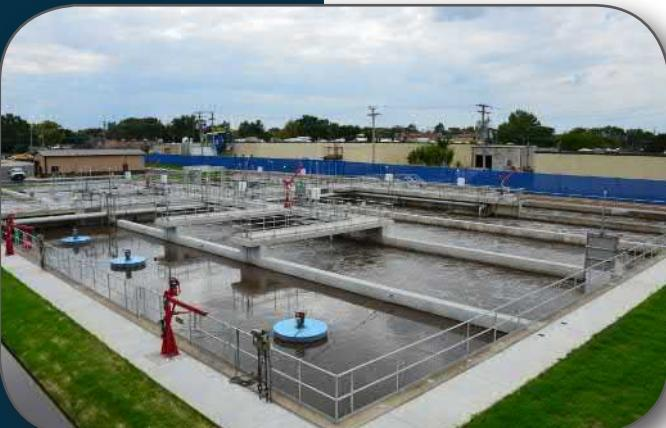
**5 FINAL CLARIFICATION AND RAS PUMPING**—Following the activated sludge process, the ML flows to the Mixed Liquor Division Box, which controls flow to each of the two final clarifiers. The clarifiers use quiescent conditions to allow the biological solids to settle from the water. Solids separated in this process are pumped from the bottom of these tanks and returned to the activated sludge process or wasted as biosolids.
