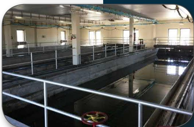
**7 DISINFECTION**—From the Parshall flume the flow continues into the chlorine contact tank. This process kills any bacteria that remains in the effluent stream. The effluent is then dechlorinated before flowing by gravity into Addison Creek.
