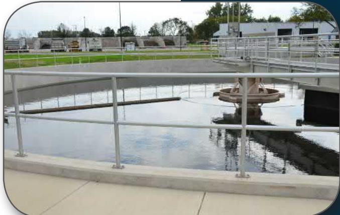
**6 TERTIARY FILTRATION**—The treated secondary effluent flows by gravity from the clarifiers to the tertiary sand filters. This process further removes suspended solids from the clarified effluent. Effluent from the tertiary filters then flows through the effluent flow metering Parshall flume.
